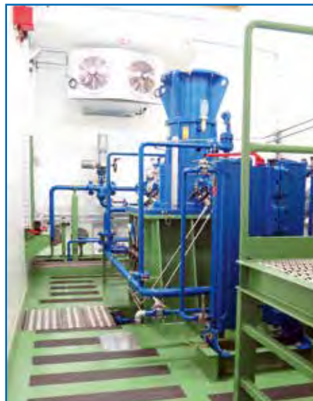
▪ Apollo high-pressure Pump Skid with vertical can-type pump
